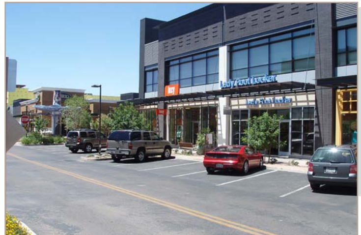
Buildings should be placed along a common streetscape with on street parking.
