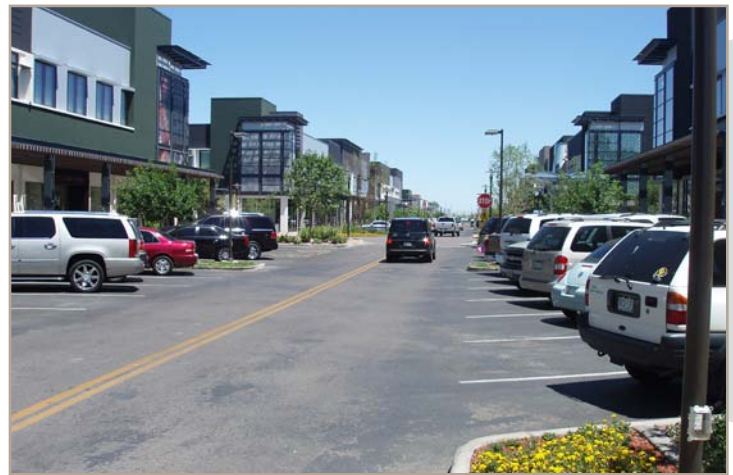
Example of changes in facade and architectural elements with a common theme.
