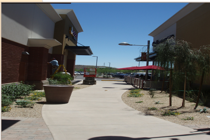
Example of a pedestrian plaza leading to a parking lot. Seating and shade should be added.
